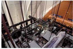
JR Clancy provided 70 counterweight sets with a loading gallery – scalable to 90 sets as required - and a computer-controlled house curtain. Clancy also provided a 450kg, steelframed fire curtain, and a house curtain on a custom hoist, with a speed of 0-115m per minute.
