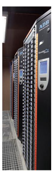
rehearsal, in which some of the lighting functions are restricted to prevent uncontrolled lights during rehearsal; performance mode, in which the system is 'locked out' to all but front-of-house lighting control; and night mode, where some of the panels are illuminated to allow cleaning staff to select house and work lighting.
