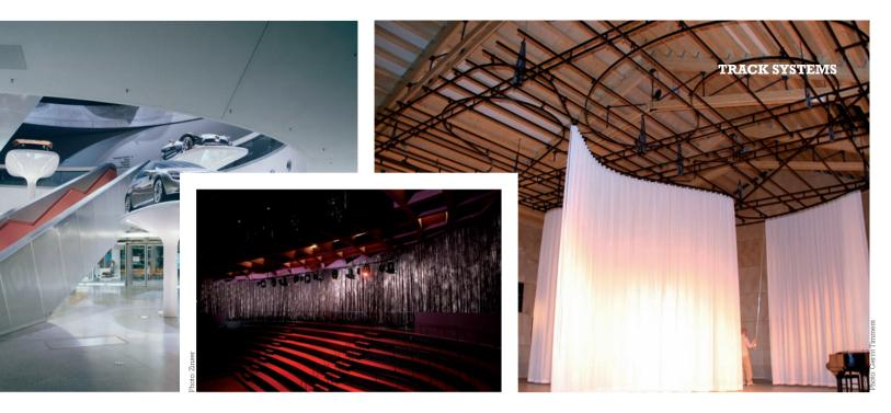
and heavy-duty systems Cargo that can handle loads up to 1200kg, yet can operate safely, quietly and reliably throughout performances. At the O.T. Theater in Rotterdam, for example, the Trumpf 95 curtain track system was combined with a light muslin textile in a complex, curved configuration to maximise the versatility of this small performance space.
