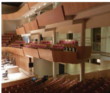
(Above and below) The view from the choir balcony shows the intimacy of the space, while the floating side balconies – with integrated reflectors – enhance resonance volume and early reflections
