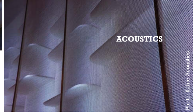
Right: The transparent metal mesh and its acoustic shelves are optimized in order to create the desired early reflection coverage in the Jinan concert hall
