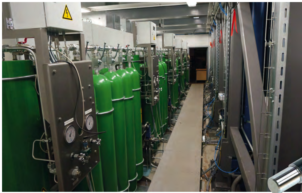
Left: The accumulator station in the venue's machine room
